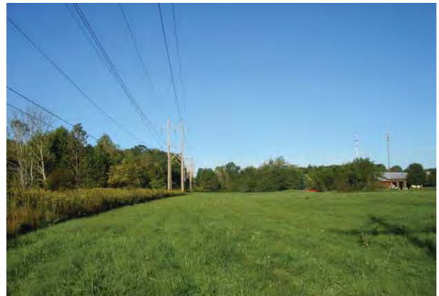
View of the south side of the Water Treatment Plant
