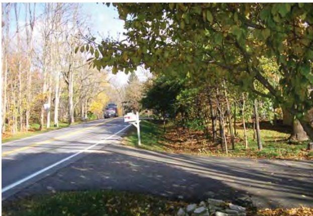
View of the existing Right-of-Way along SR 315
